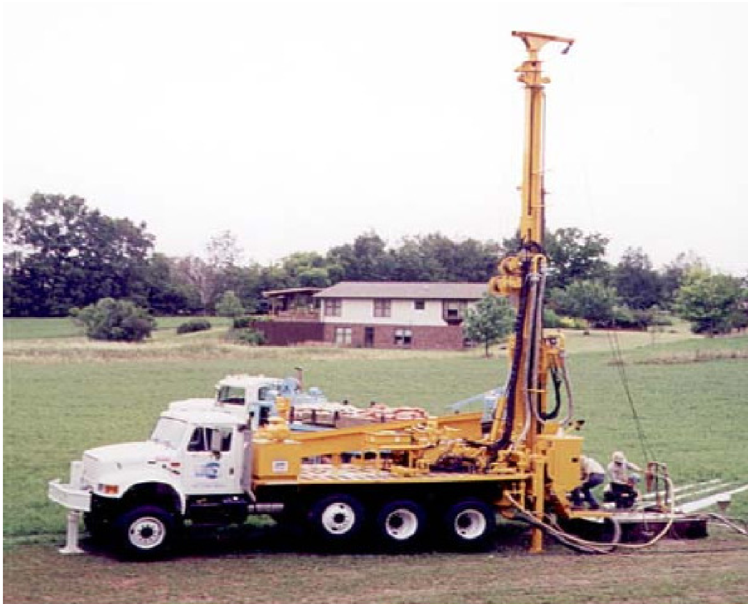
Figure 7: A typical borehole drilling rig
