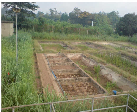
Plate 1: Pilot Scale Reedbed showing the irrigation pipe and the sludge drying beds.
